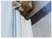
The mast profiles are fitted with rubber seals to to prevent scratching and to make the area entirely waterproof. The height can easily be adjusted.
